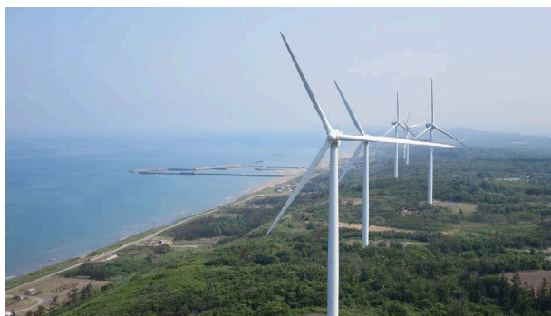
Oga is an ideal site for wind power generation, with average annual wind velocity exceeding 6 m/s at many points. (Oga wind power plant)
