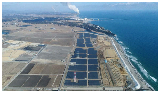
Second-phase construction; Haramachi Higashi solar power plant
