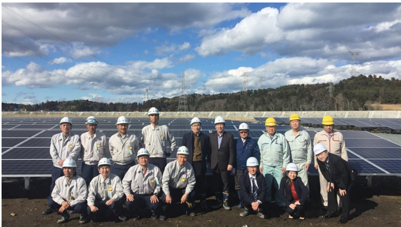
Our affiliate conducts panel inspections at periodical local meetings. (Second-phase construction; Haramachi higashi solar power plant)
