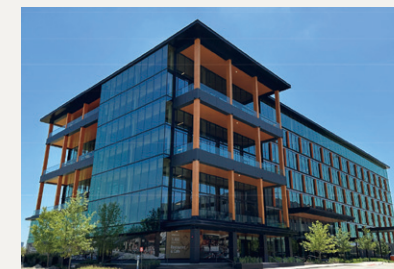
7-story wooden office in Dallas
