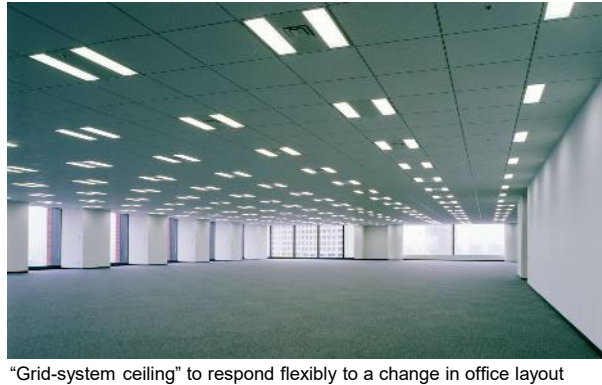
“Grid-system ceiling” to respond flexibly to a change in office layout
