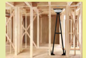
Vibration control unit "MIRAIE" for detached housing, developed from the experience of two major earthquakes
