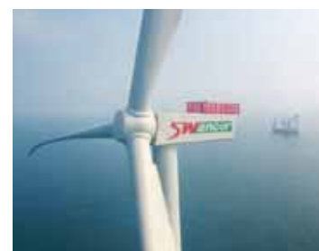
Offshore Wind Turbines in Zhunan
