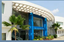
Setup manufacturing unit in MEPZ-SEZ Chennai
