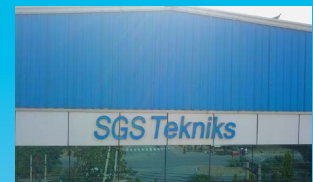
Setup manufacturing facility in Manesar
