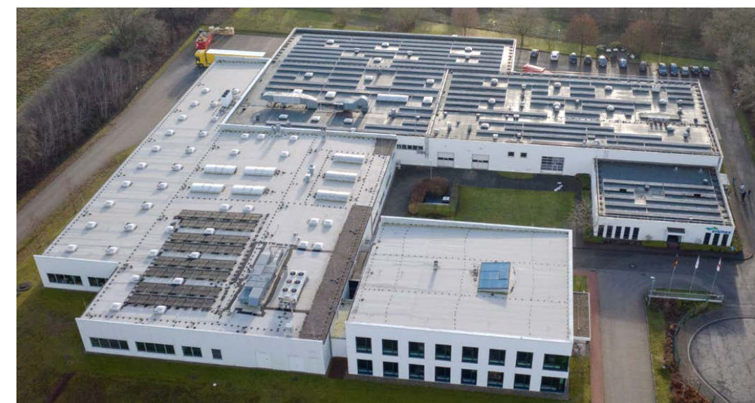
The reagent production facility uses electricity generated by its own solar panels on the facility roof.
