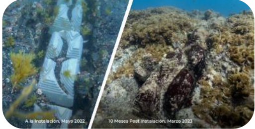
Protection of submarine cables with concrete blocks with ecological design
