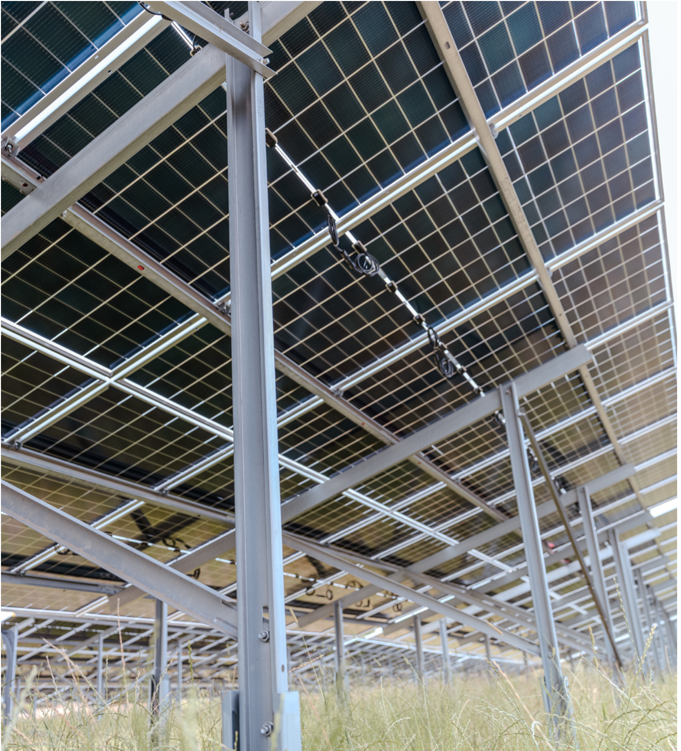
MagiZinc steel profiles are used in solar panel mounting structures.
