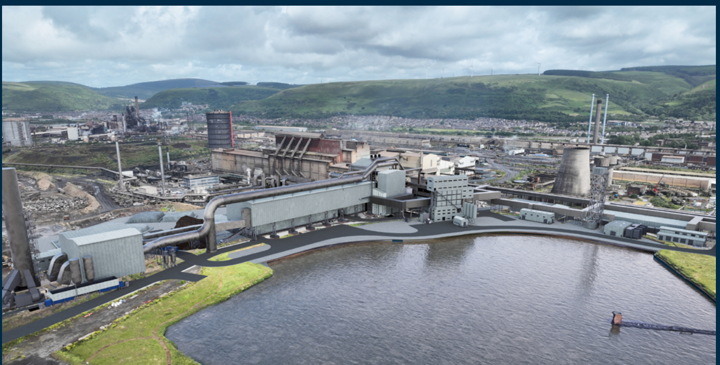
Artist's impression of the Port Talbot site showing the electric arc furnace (centre) due to be installed in 2026.
