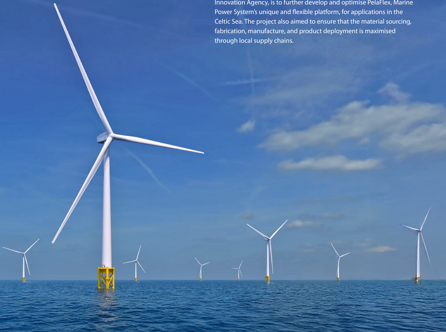
Floating offshore wind installation in the Celtic Sea.
