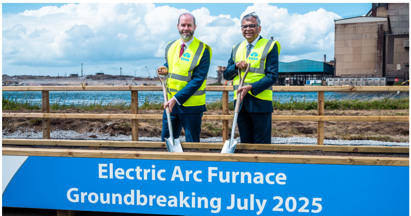
Jonathan Reynolds, Secretary of State for Business and Trade and Mr N Chandrasekaran, Chairman Tata Steel at the groundbreaking ceremony for the new EAF in July 2025.
