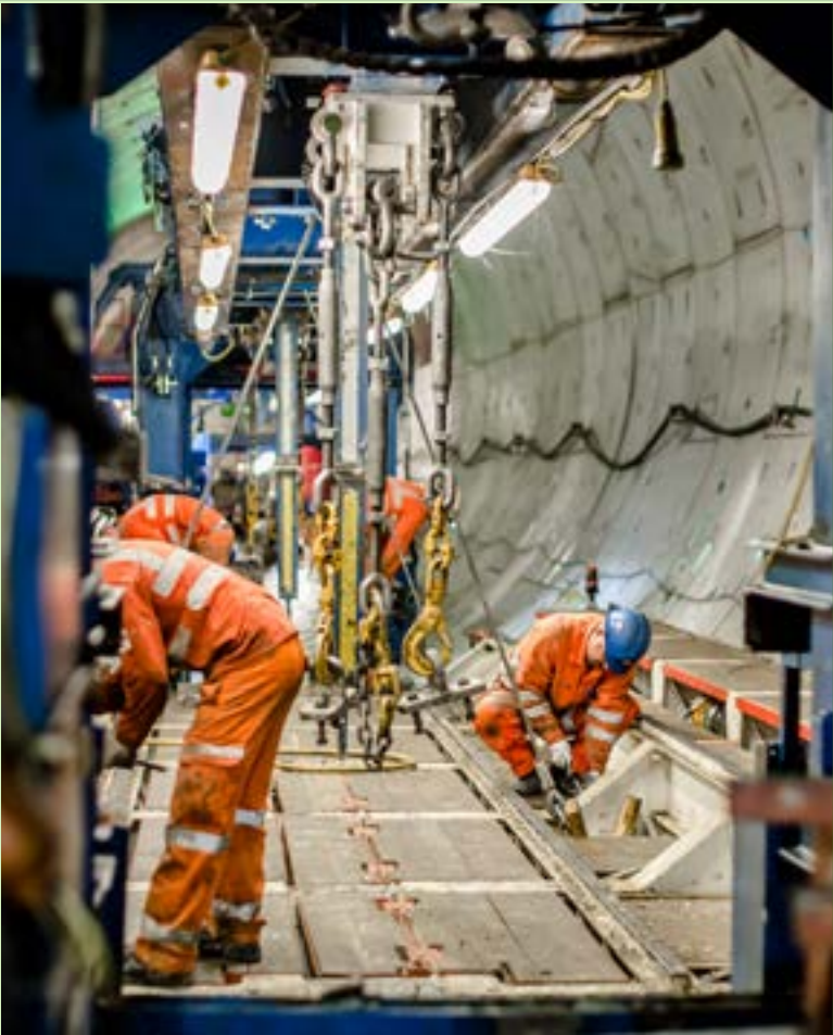
Construction of the Lee Tunnel, part of the London Tideway Tunnel Network
