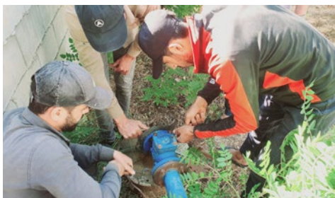
Repairs to water supply facility in Idlib, Syria
