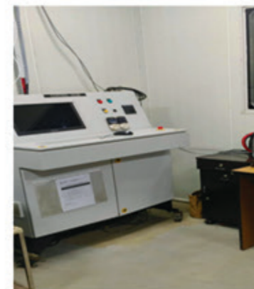
Master Controller for Combined System Test
