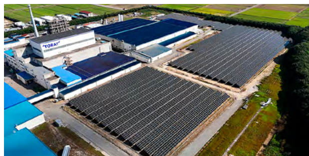
Ishikawa Plant Solar Power Generation Facility
