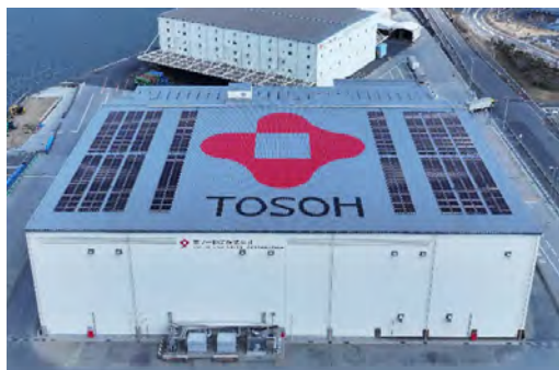
Integrated Rinkai Logistics Center Building A
