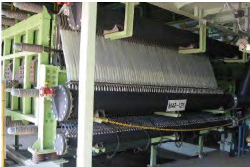
New caustic soda electrolyzer
