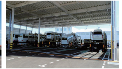
Installation of a roof over the loading area
