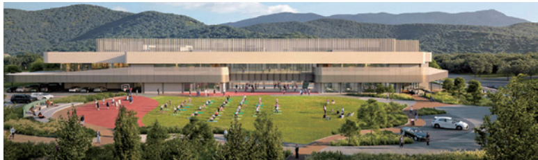
Completion image of the Toyota Sports Center Gymnasium 1
