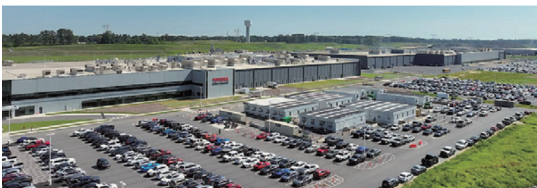
Automotive battery plant in North Carolina, the U.S.
