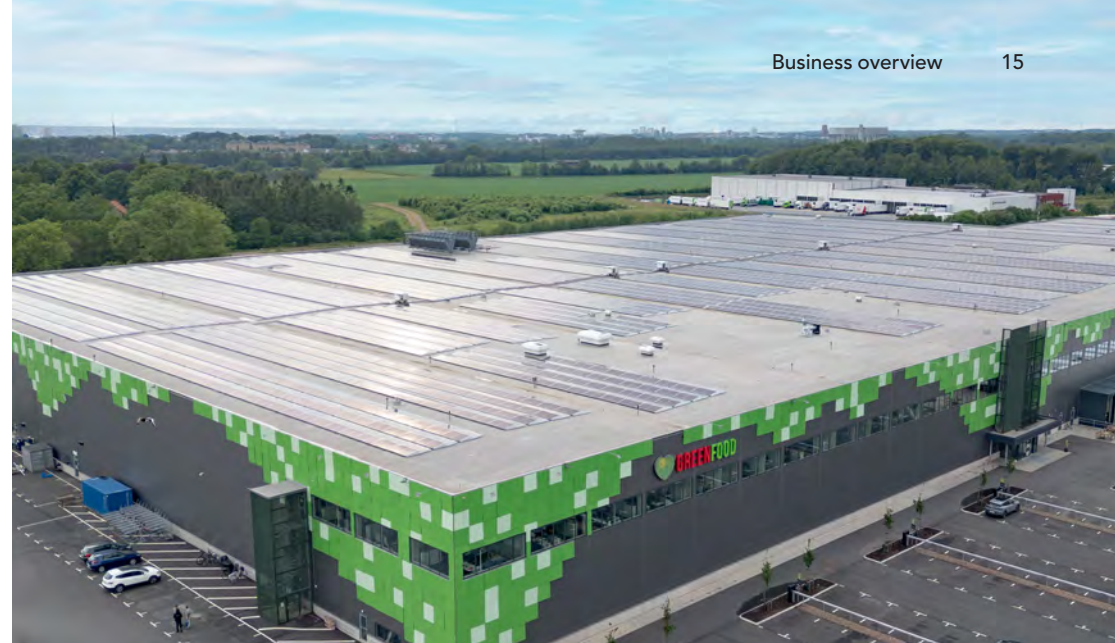
6,916 solar panels, producing 3.5 million kWh per year, were brought online. They cover 17,800 m 2 of Greenhouse's roof area and generate 20 percent of Greenfood's electricity needs, reducing our CO 2 emissions by 150 tons per year.
