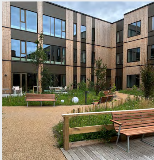
Altiden's Fribo Greve nursing home, with 75 beds, opened in June 2023.
