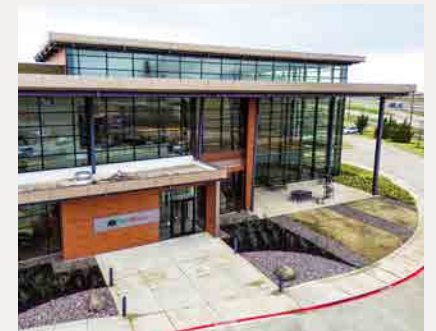
TreeHouse Foods' Coffee Center of Excellence located in Northlake, Texas.
