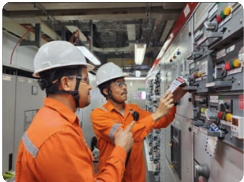
Energy isolation through the lock-out process
