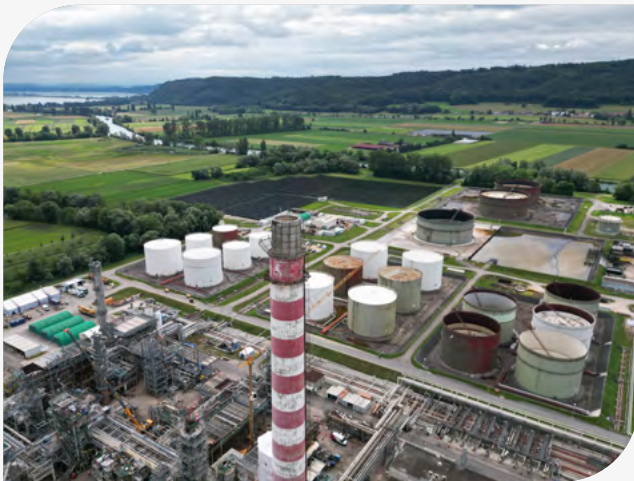
Residual heat can be used by local communities to reduce emissions.
