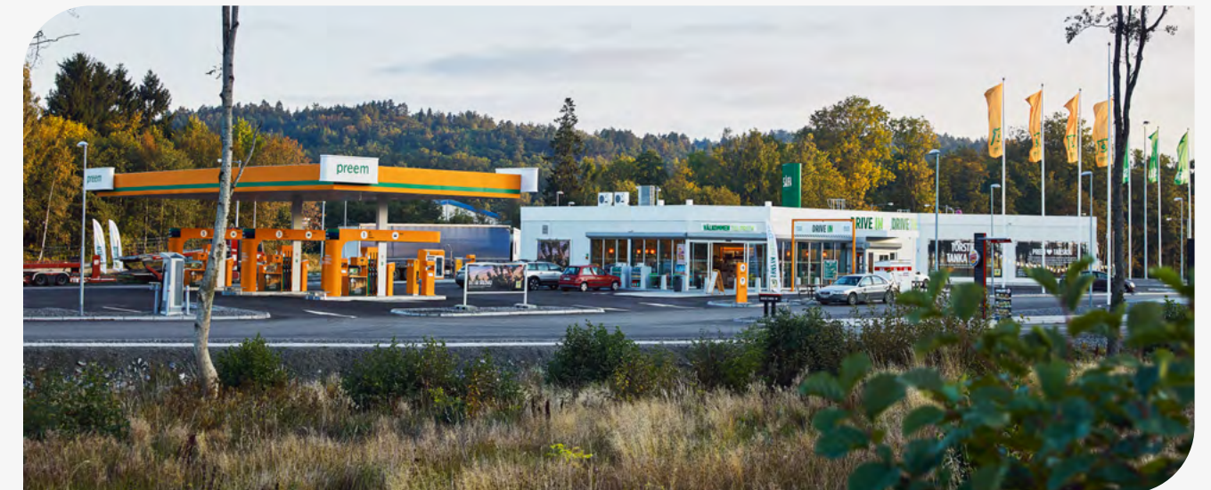
The first Nordic Swan Ecolabel-certified HVO100 enables customers to reduce their fuel emissions.
