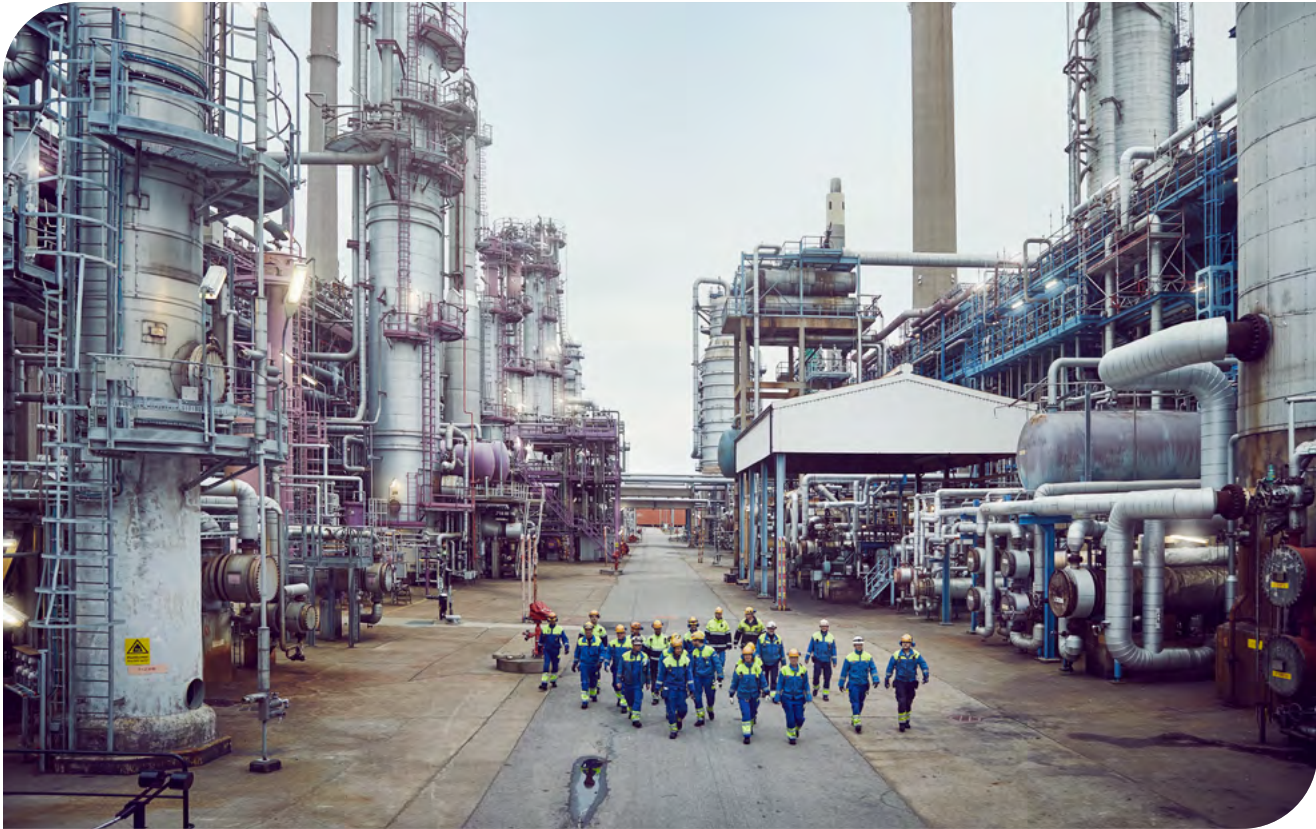
Lysekil is the last major refinery built in Europe (1975).
