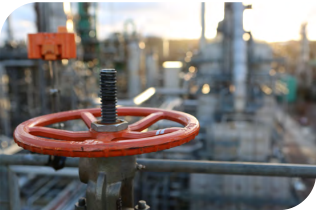
VAROPreem investigates and reviews the causes of any leak to avoid similar incidents from occurring in the future.
