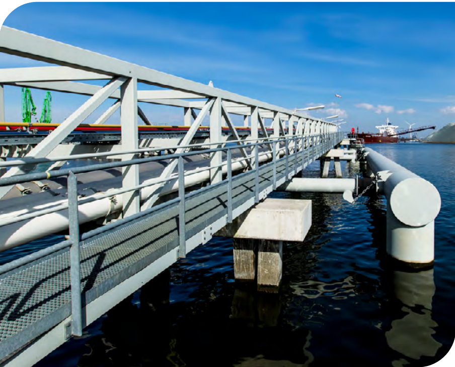
Jetty and pipeline infrastructure at VAROPreem’s Amsterdam terminal in the Netherlands.
