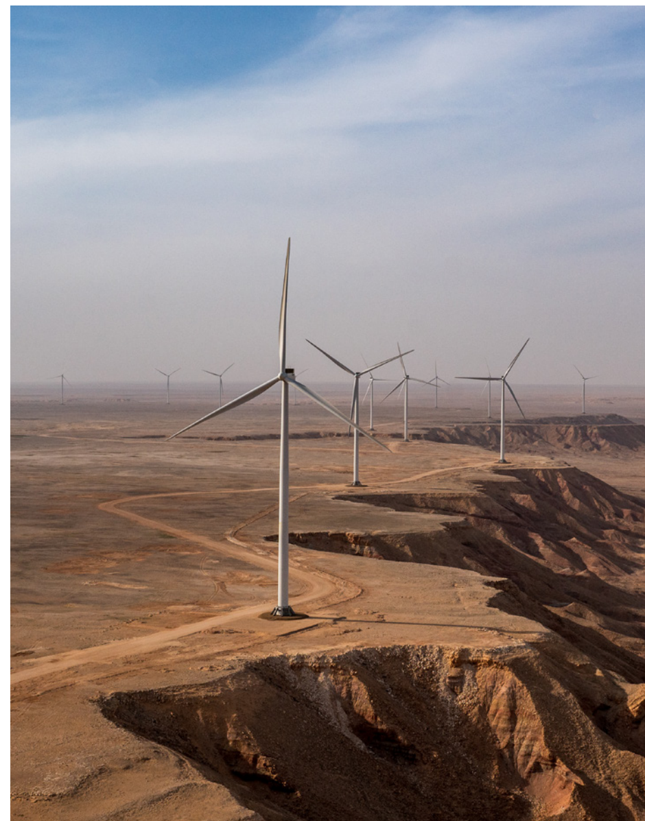
→ The Dumat Al Jandal wind park in Saudi Arabia features 99 V150 4.2 MW turbines. With a total capacity of 415 MW, it is the country's first utility-scale wind park.
