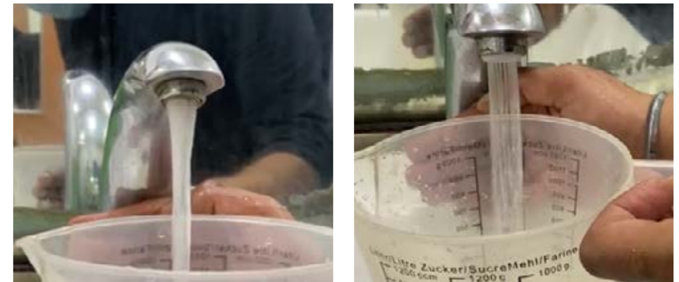
Overall, 5% water saved due to eco nozzle usage in water taps that reduces consumption from 6 lit/min to 1.5 lit/min
