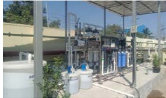
20% water reduction- Domestic water is treated & used for process at plant avoiding purchase of DM water- 15KL/day
