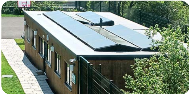
Castlefell School Solar panels installed
