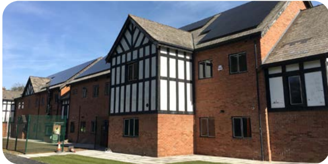
Cheshire Hall School Solar panels installed
