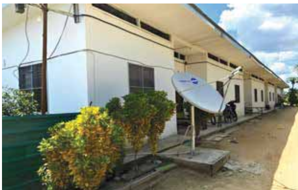
TV antenna set-up in labour quarters
