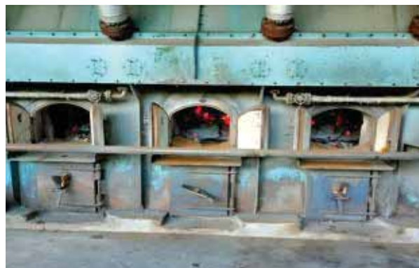
Using palm fibres as fuel for palm oil mill's boiler to generate steam for electricity
