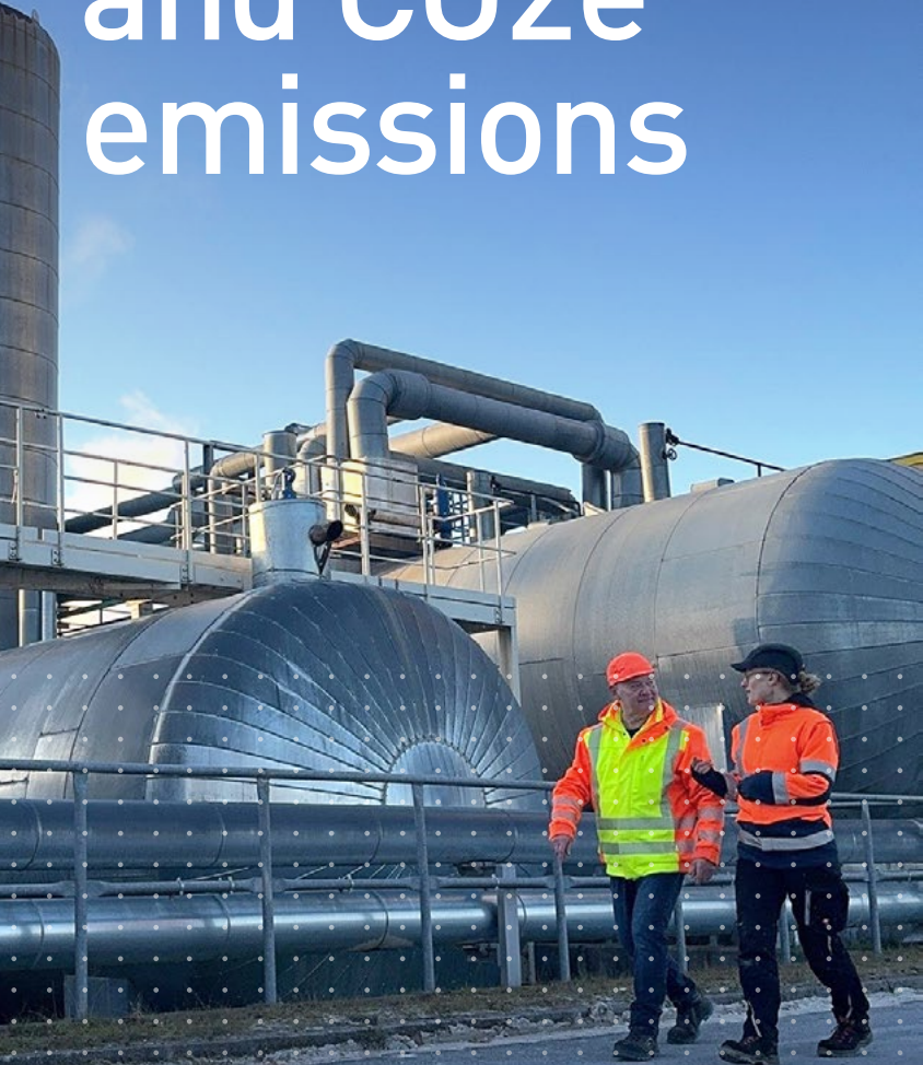
Inspection of autoclave insulation at the Brück plant, Germany.
