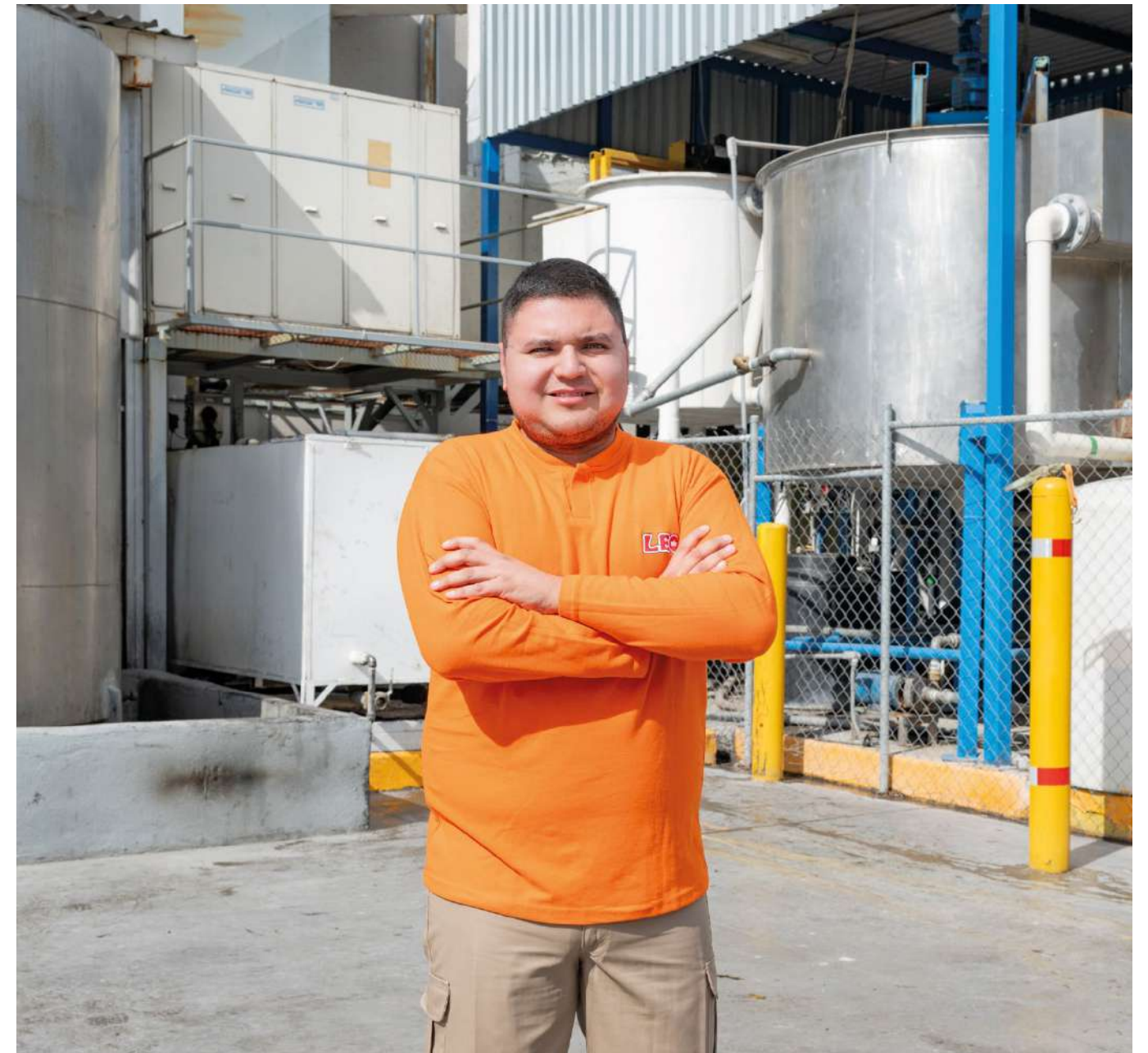
Our Wastewater Treatment Plant (WWTP) at the Monterrey Plant helps us to manage this resource responsibly.
