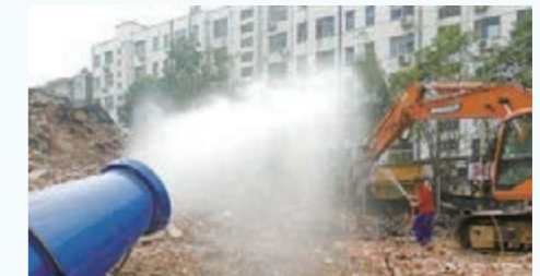
Site Dust Control: Fog Cannon
