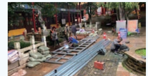
Framework Platform Welding
