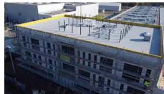
Expansion of the production and storage area by 12,500 m 2 in Ilawa
